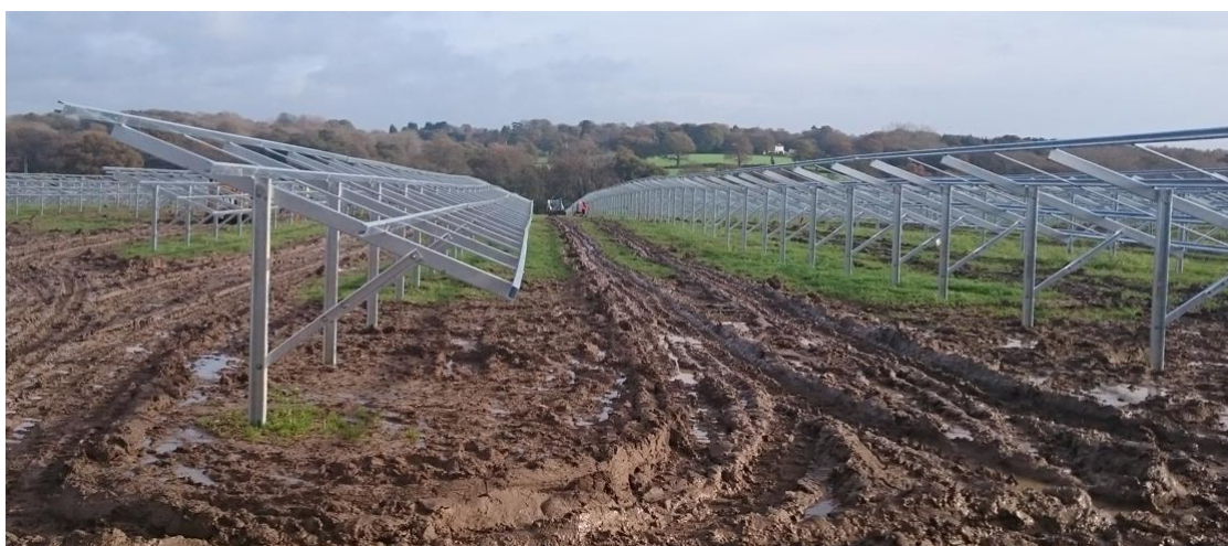
Inserts 2 and 3: Inter-row Ground Restoration
